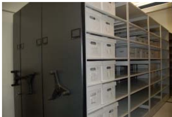
The beautiful new Spacesaver shelves installed!
