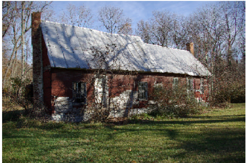
Two structures conjectured to be slave cabins in southern Anne Arundel County. One was moved and connected to the other in order to create a larger house. While actually covered in wooden weatherboard, the houses were sheathed in asphalt paper with a brick pattern in order to make them look like they were built with better materials than they really were.
