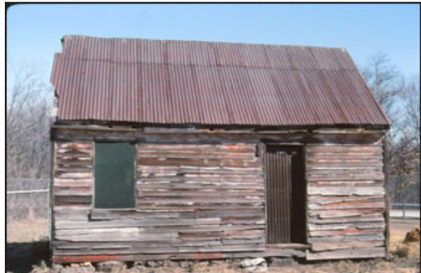
The slave quarters at Grassland prior to restoration in 1994.
