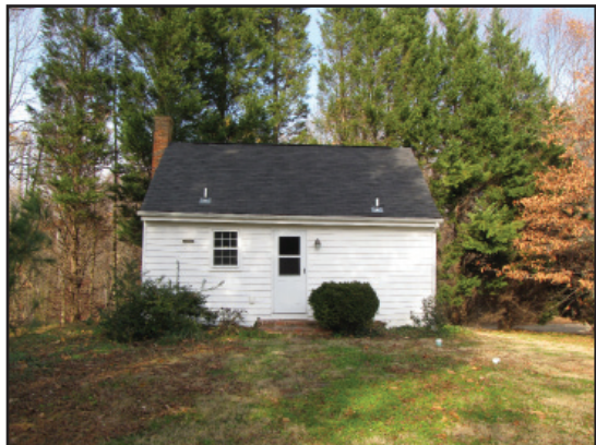
The servant's quarter, located less than 400 feet from the main house.
