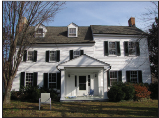
Main facade of Batchelor's Choice shows the original 3-bay wide portion on the left, and the taller 2-bay wide ca. 1840s addition on the right. The doorway and porch were added in the 1840s.
