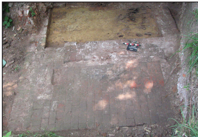
One of the massive brick chimney bases uncovered in the cellar of the mansion ruins.
