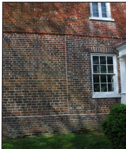
Brick Bonding Pattern on the First Floor
