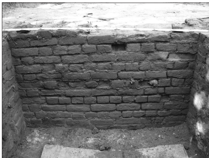
FIGURE 9. English bond used in bulkhead entrance.
