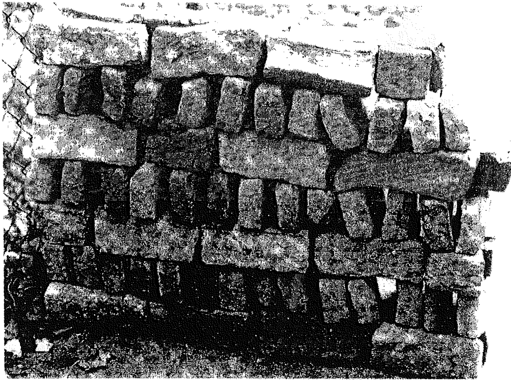
FIGURE 10. Reconstruction of the interior of the firebox (lacking mortar and parging).
