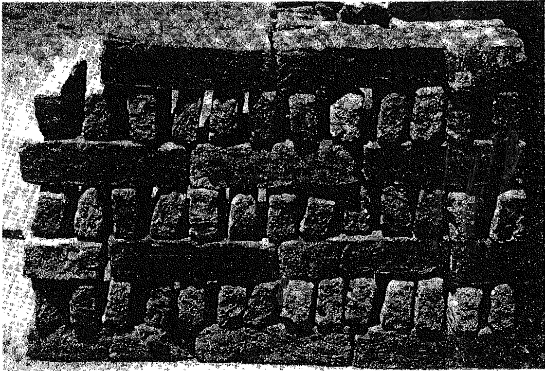
FIGURE 8. Reconstruction of the exterior of the firebox (lacking mortar and scribing).
