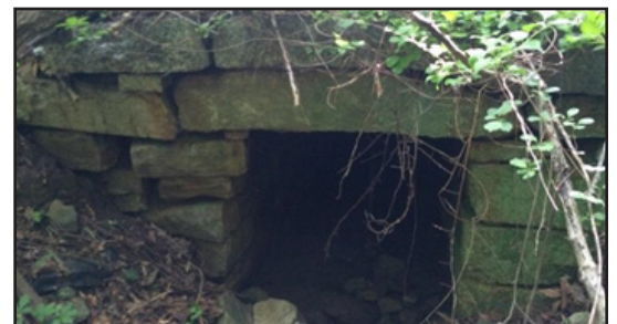
Dressed Stone Culvert, likely Part of the Original 1838-1840 Construction
